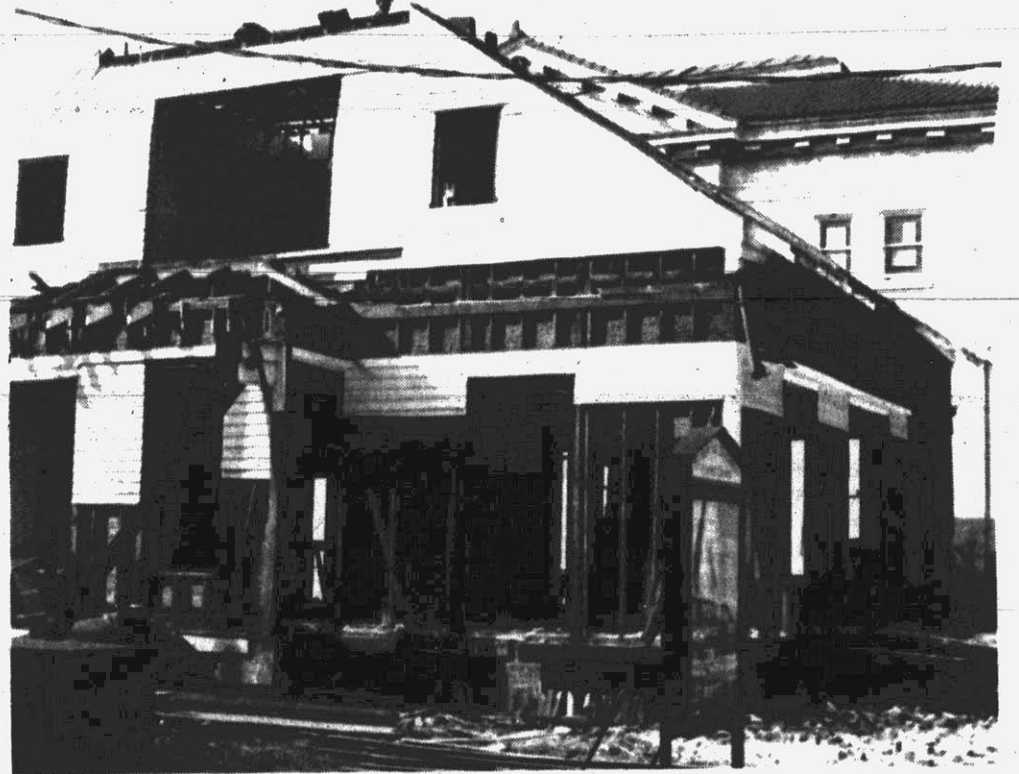
PARSONAGE . . . being dismantled at Sycamore Hill Baptist Church.
