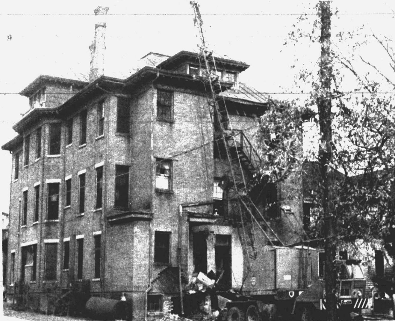
THE VINES HOUSE . . . which has sheltered over 30,000 persons, faces its last days.
