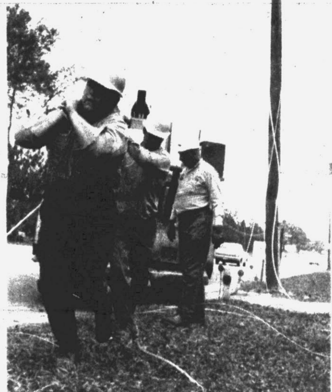
WORKING HARD . . . to get power restored, Greenville Utilities Commission employees pull wire along Memorial Drive after wires burned down. (Reflector Photo by Tommy Forrest)
