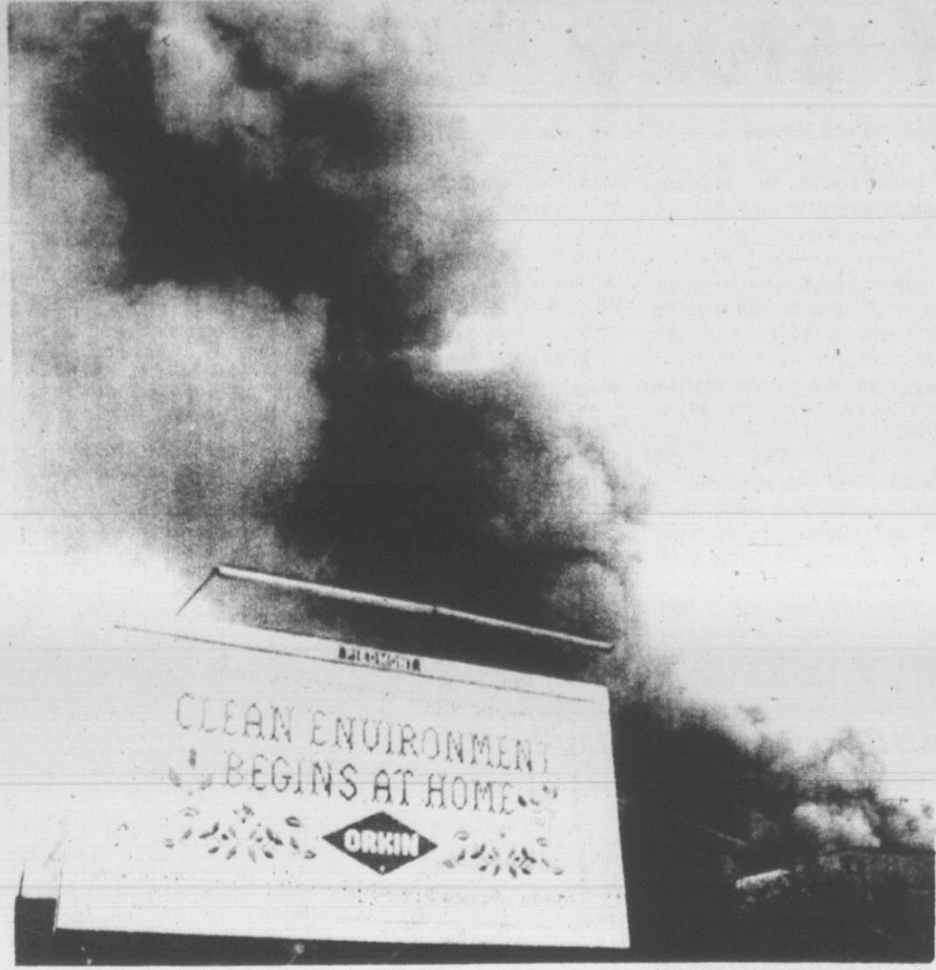
BILLOWING SMOKE from a downtown Greensboro fire formed an ironic backdrop Sunday for a billboard. Firemen brought the fire under control just after dark, limiting damage to a White Cross Pharmacy. For several hours earlier however, firemen feared the fire would spread to other firms along the city's main street. (AP Wirephoto)
