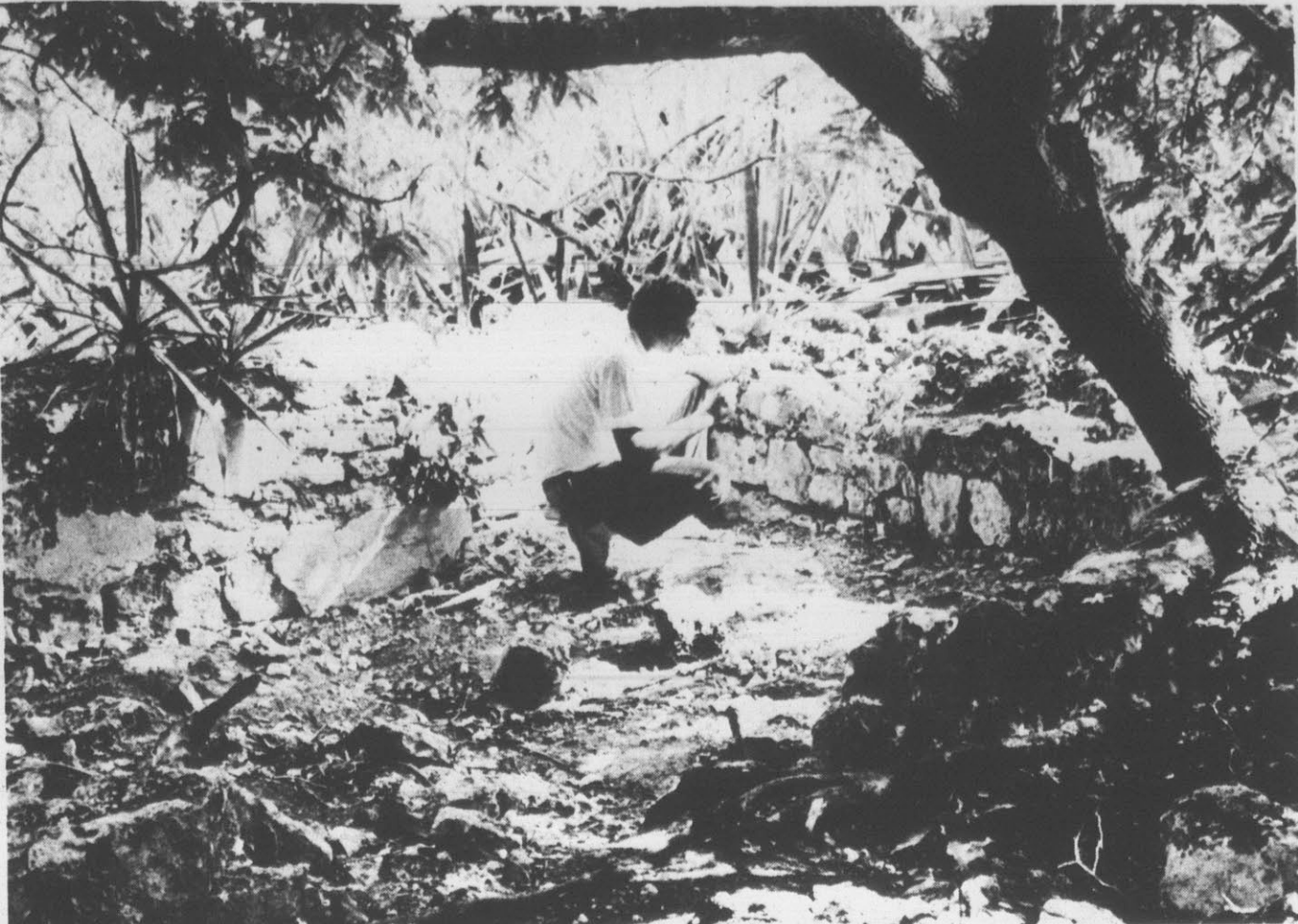
STANLEY BROWN looks over the ruins of one of the buildings on Indian Key (Fla.), once infamous as
