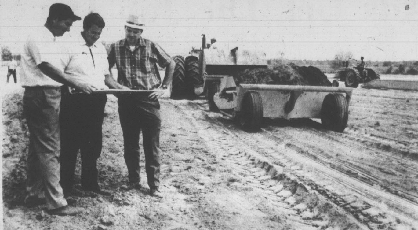
Shaping It Up
