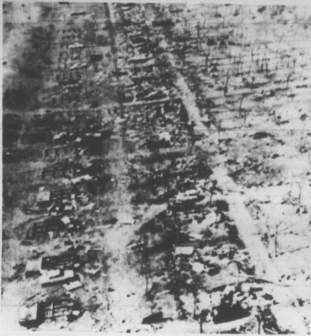
CAMP SITE RAZED BY ITALIAN CYCLONE — Ruined bungalows and flattened trees mark the swath a cyclone cut through this devastated camp site north of Venice, Italy, late
