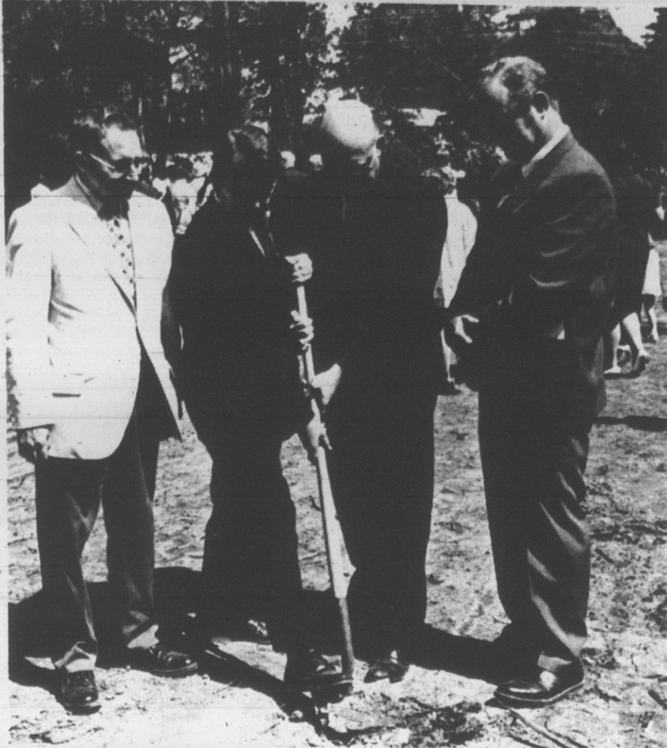
GROUND WAS BROKEN yesterday on the planned site for Red Oak Christian Church's new building. Four who participated in the service were (left to right) J.T. Manning Jr., the Rev. Kenneth Moore, Dr. Charles E. Dietze, and James Sydney Allen.
