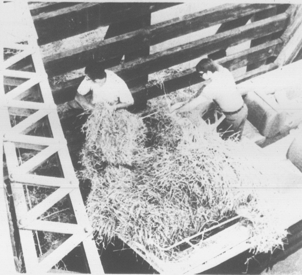
BARRIER AT GRIMESLAND. . . A barrier was placed at the bridge in Grimesland to prevent any further flow of oil. Above a workman from the N. C. Department of Water & Air Resources throws hay into the river as a Greenville volunteer Nat Van Nortwick (right) assists. (Reflector Photos by Tommy Forrest)
