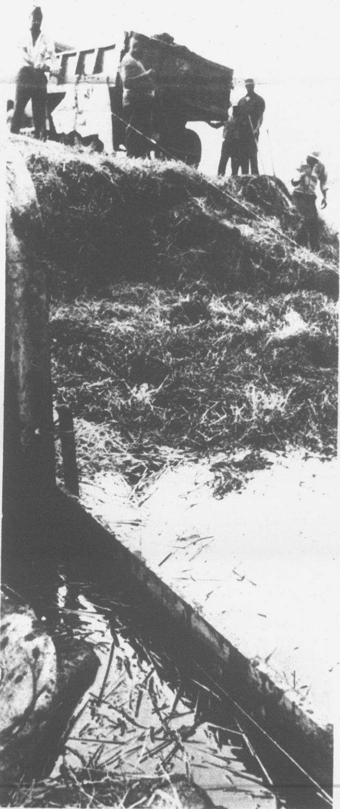
GREASY PROBLEM. . . Workmen from the Greenville Utilities Commission retrieve soaked hay from the mouth of the town creek, trying to curb the flow of the oil into the Tar River.
