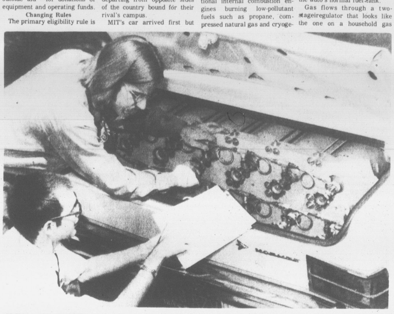
CLEAN AIR RACER — Jim Henry, 21, of San Francisco and Greg Kendall, 21, San Gabriel, check valves of bank of 12 Scuba tanks mounted in trunk of their car. Tanks contain compressed natural gas — power source for Cal Tech's race entry. (UPI Telephoto)
