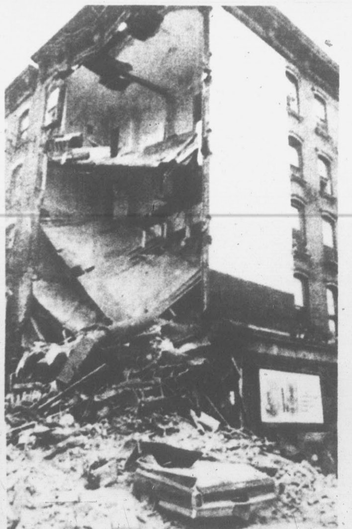
BUILDING COLLAPSES... when vehicle crashes into it. (AP Wirephoto)
