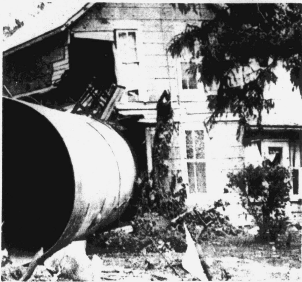
HOME DAMAGED . . . section of Crescent City, Ill. after series of ex-tank car protrudes from a house in pliosions. (AP Wirephoto).
