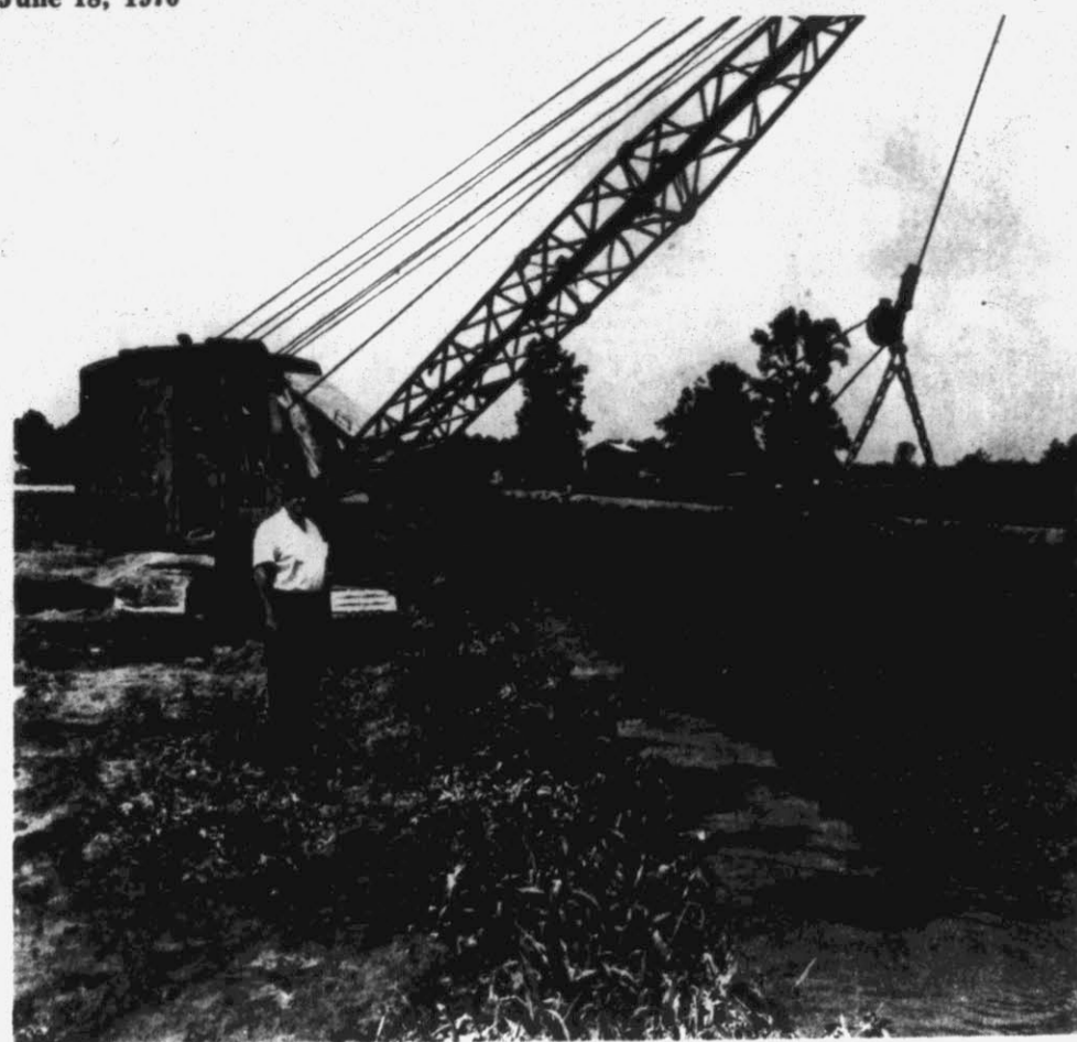
MAINTENANCE CLEAN-OUT — Edgar Warren and his neighbors recently did a maintenance clean-out on a two-mile stretch at the upper end of the Atkinson-Clark canal. Approximately 33 property owners participated in the project. The Soil Conservation Service furnished technical assistance to the group. (SCS Photo by Elmer Bland)
