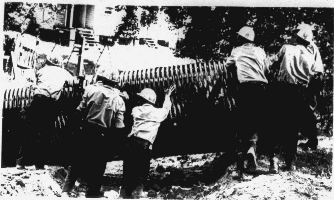
IT TAKES MANPOWER... as well as machines to do a big job. Here, several city employees assist in positioning a large pipe being installed in the drainage project now being completed in the
