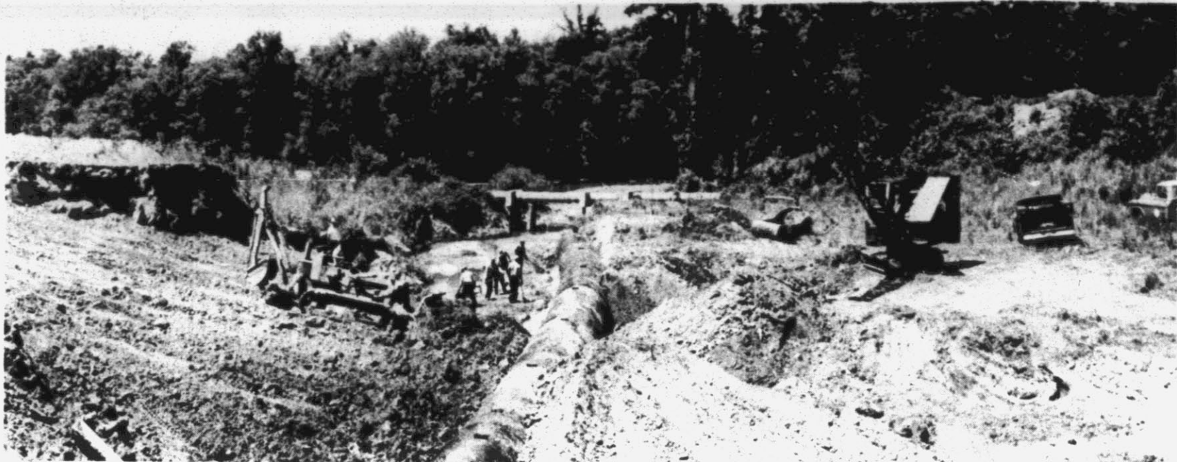
TOWN CREEK GOES UNDERGROUND — Workmen this week are putting in 240 feet of 78-inch drainage pipe at Town Creek between First Street and the river in the Shore Drive park. The work will eliminate an erosion problem at the east end
