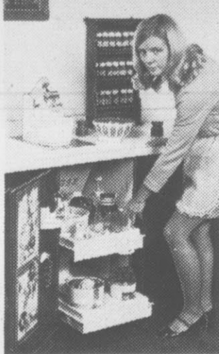
BUILT-IN FOOD preparation center installs in a kitchen cabinet, and comes with a variety of cooking aids and appliances, operated by its own power module. It's Ronson's "Foodmatic."
