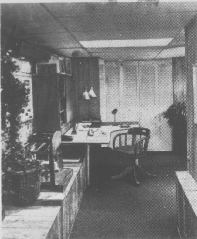
HISTORIC HOME , BUILT IN 1856, GETS a roomier, remodeled basement with help of modern building materials. Studio area preserves original brick wall, left, while other walls, ledges are sheathed in Early American siding. Bi-fold metal doors conceal gas and electric meters, and ceiling system covers network of pipes. Indoor-outdoor carpeting helps combat dampness. Doors, siding by U. S. Plywood; Weatheron carpeting, ceiling by Armstrong.
