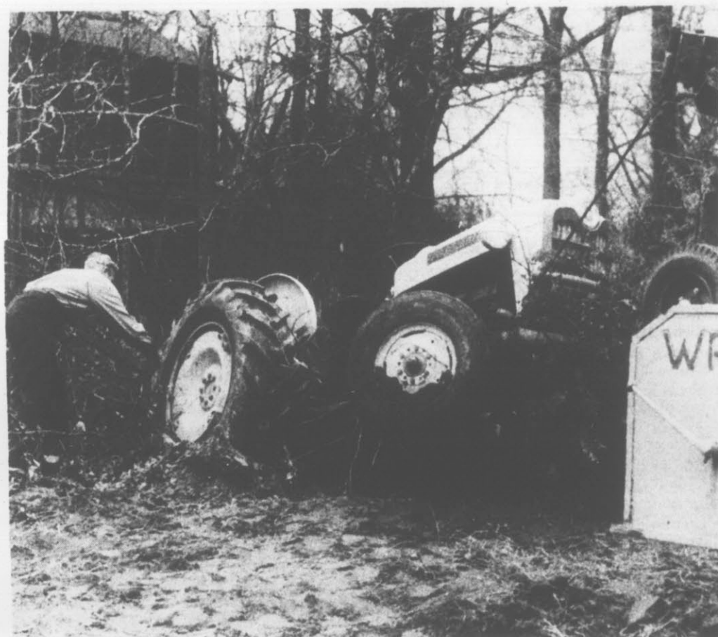
DEATH SCENE . . . Workers remove tractor from six-foot deep ditch where man was killed yesterday.
