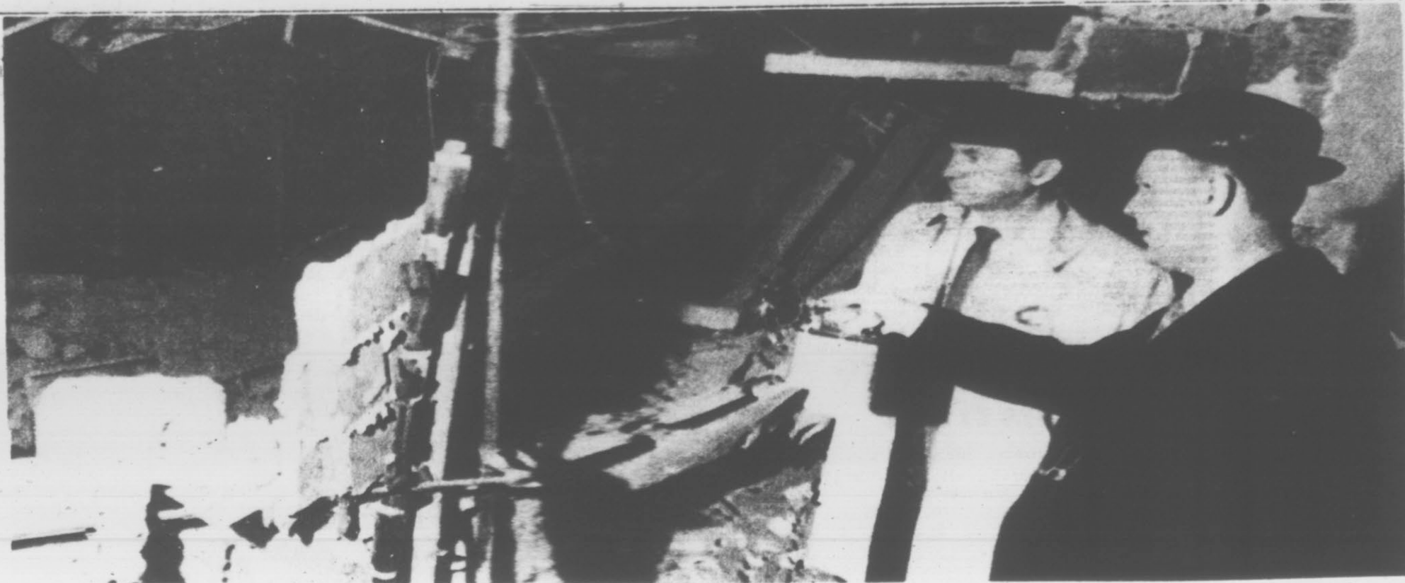
EXPLOSION DAMAGE — New York City bomb squad official sines light on damaged area of interior of building at 150 E. 42nd St. in Midtown Manhattan this morning. (AP Wirephoto)
