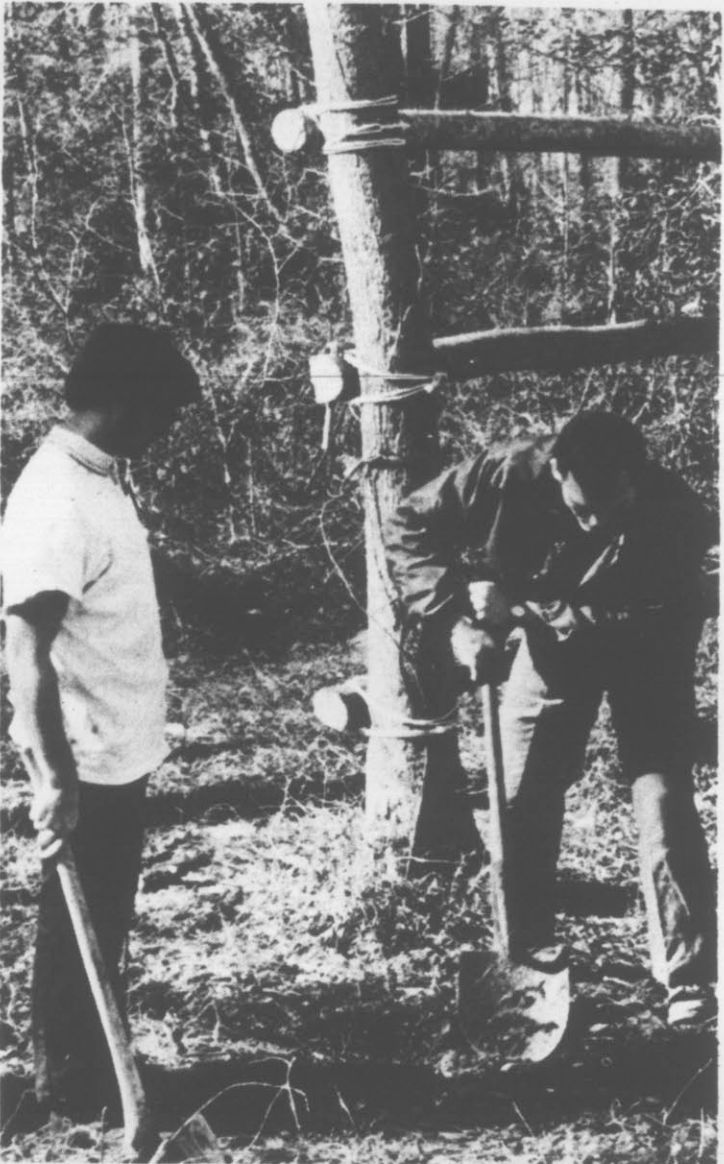
TAKING TURNS . . . in cutting roots and shoveling, two volunteers combine their efforts to dig a small drainage ditch in the lower part of the course.
