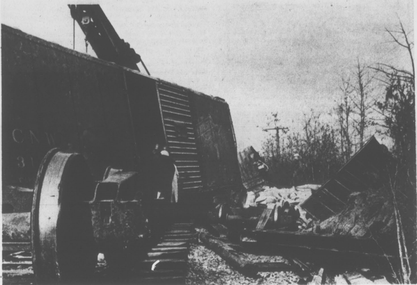
Clearing The Tracks
