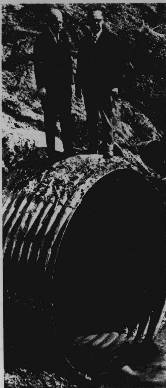
FORNES RUN SOLUTION . . . Mayor Frank Wooten (L) and city engineer Charlie Holliday stand on the large new 96 inch pipe that now carries Fornes Run water under the Norfolk Southern Railway. Flooding problems should be lessened.
