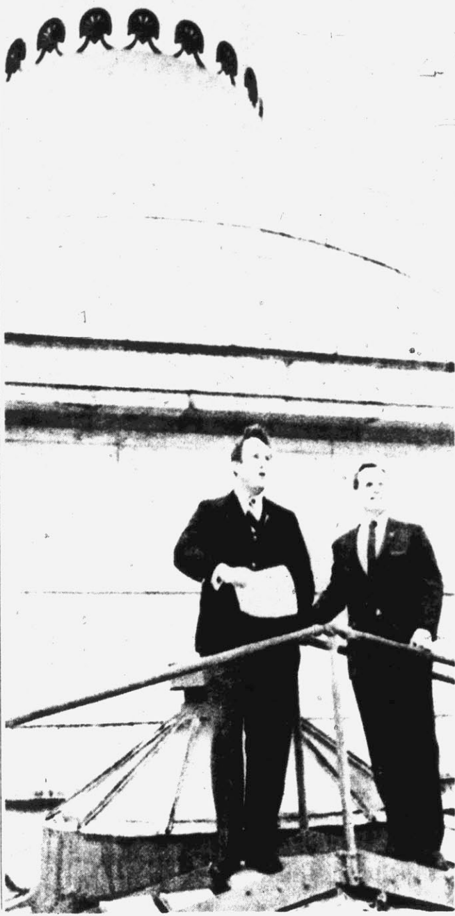
INSPECTS CAPITOL—Gov. Bob Scott (left) and Dr. H.G. Jones, director of the N.C. Dept. of Archives and History, are shown on roof of 129-year-old Capitol. (AP Wirephoto)
