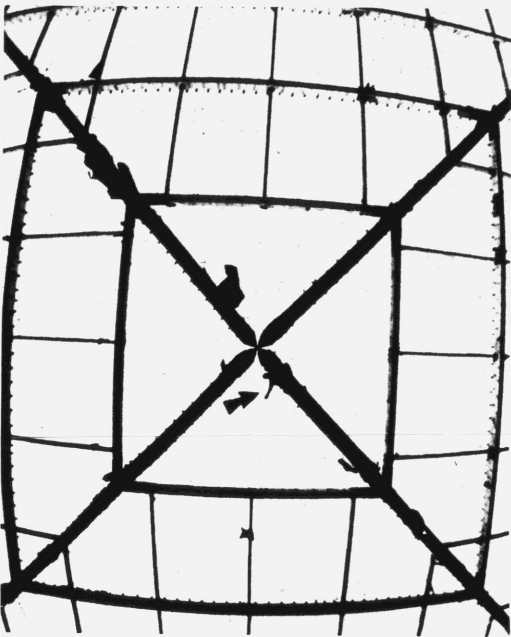
THAT'S A MAN UP THERE—A steeplejack waves with outstretched arm (arrow) from center of the huge wooden roof structure of the Shippensburg, Pa. State College new field house.
