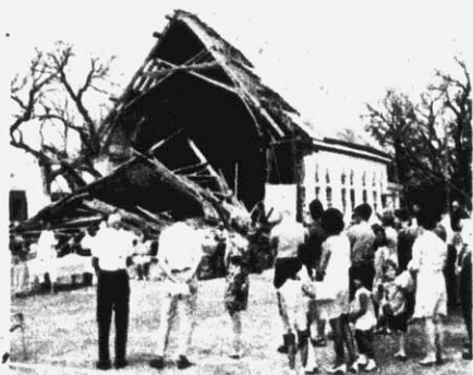
Gulf church—now rebuilding
