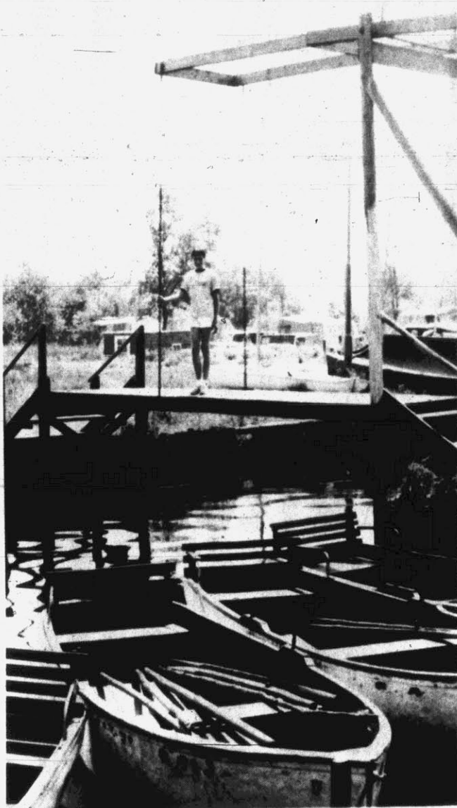
THE LEVEL . . . of the reclaimed land, called polder, is so low that drainage canals are everywhere. Here is a one man bridge which may be raised by hand.
