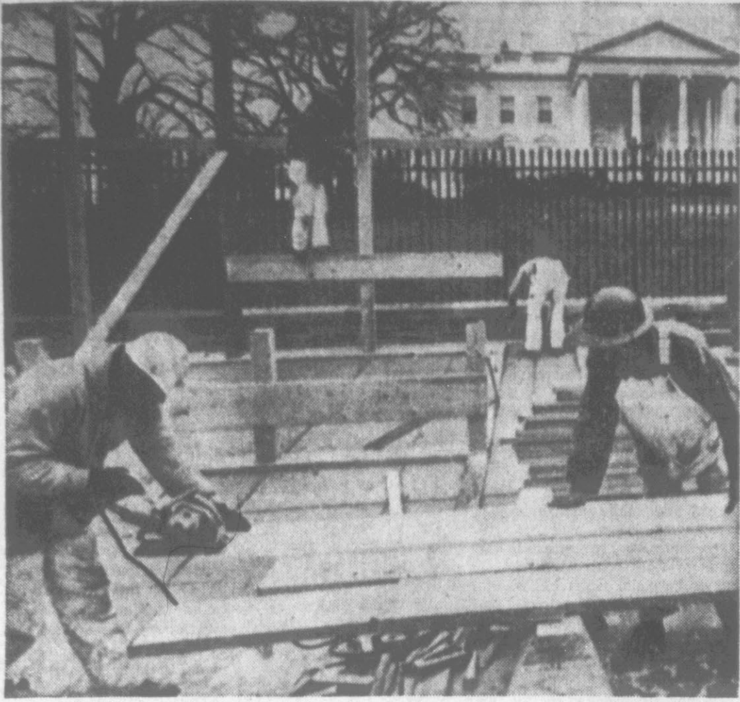
BUILDING A VIEWPOINT — Workmen construct stands on Pennsylvania Avenue in front of the White House for the Inaugural Parade on Jan. 20. Richard Nixon is to view the Parade from this area after he is sworn in as President. (AP Wirephoto)
