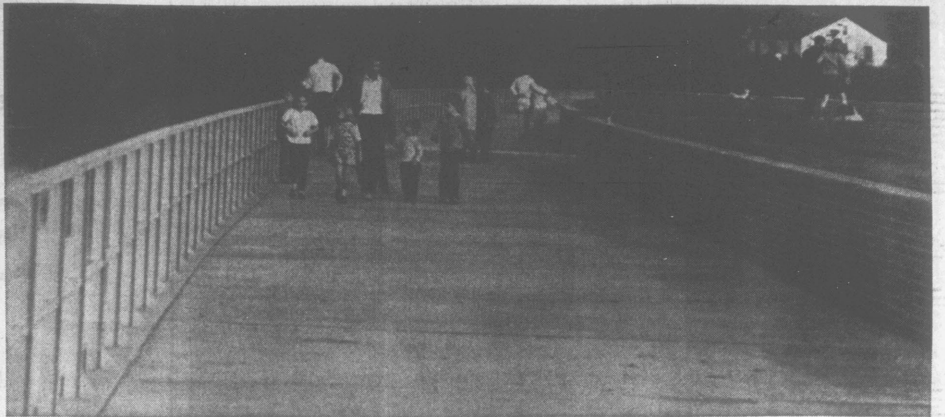
NICE DAY FOR A WALK — Greenville's recently completed esplanade atop the retaining wall on the river bank proved a popular spot yesterday as balmy weather prevailed here. The walk is built above the 1,600 foot long steel piling wall which raised the area from Greene Street to Side Street above the flood plain. A winter grass planted between First Street and the wall has turned the area into a sea of green. (Reflector Photo by Tommy Forrest)
