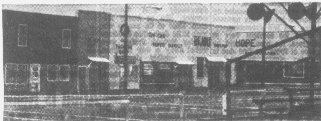
DEMONSTRATION VILLAGE . . . Mock realistic training in riot control procedures at Fort Gordon, Ga., used for
