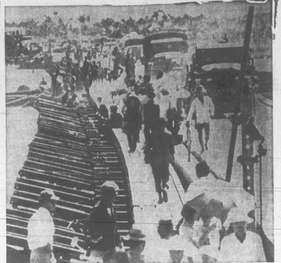
BRIDGING SAIGON WITH THE MEKONG DELTA — Civilian and military traffic flows across a pontoon bridge constructed by U. S. and Vietnamese engineers to span the Vaioe Oriental River, a tributary of the Saigon River, at Ben Luc, southwest of Saigon. The temporary
