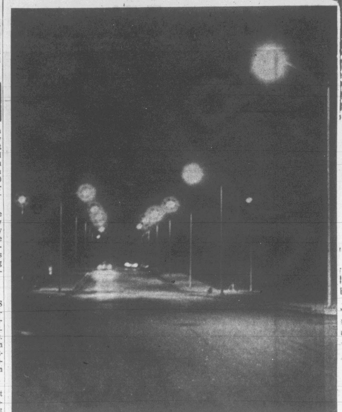
A PREVIEW . . . Greenville residents can get a preview of things to come by riding down Second Street, between Colaniche and Pitt at night. That roadway has been paved — complete with curb and gutter — and mercury vapor lighting installed as part of the Shore Drive Redevelopment project now under way in the area. When completed, all streets in the project area will look similar to the Second Street section. (Reflector Staff Photo)
