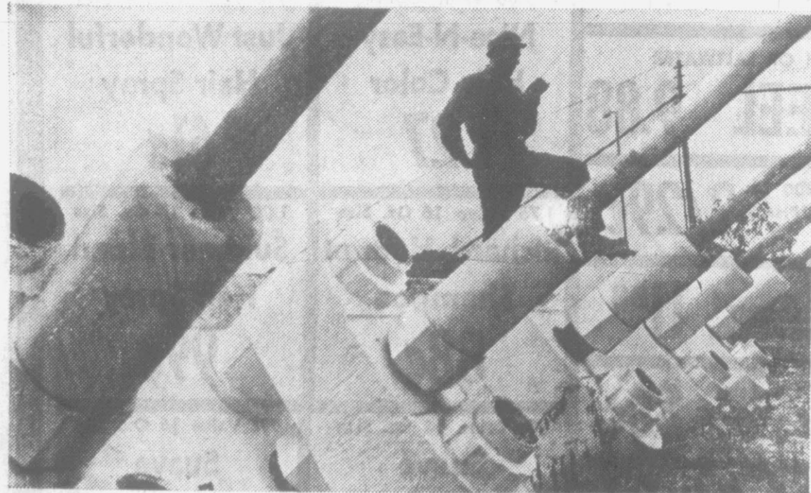
A workman stands on an anchor block unit supporting one of the three towers which suspend the triangular platform.
