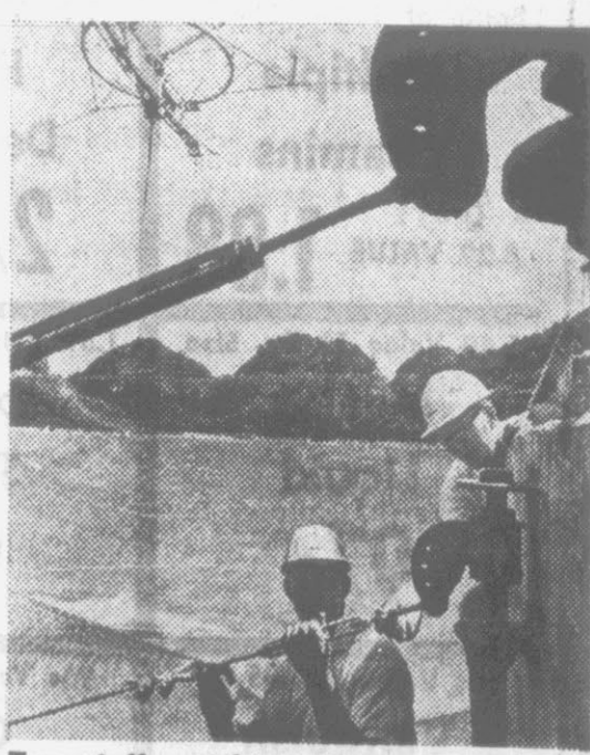
Two staff members check the linkage on the mesh-supporting cables above the reflector.
