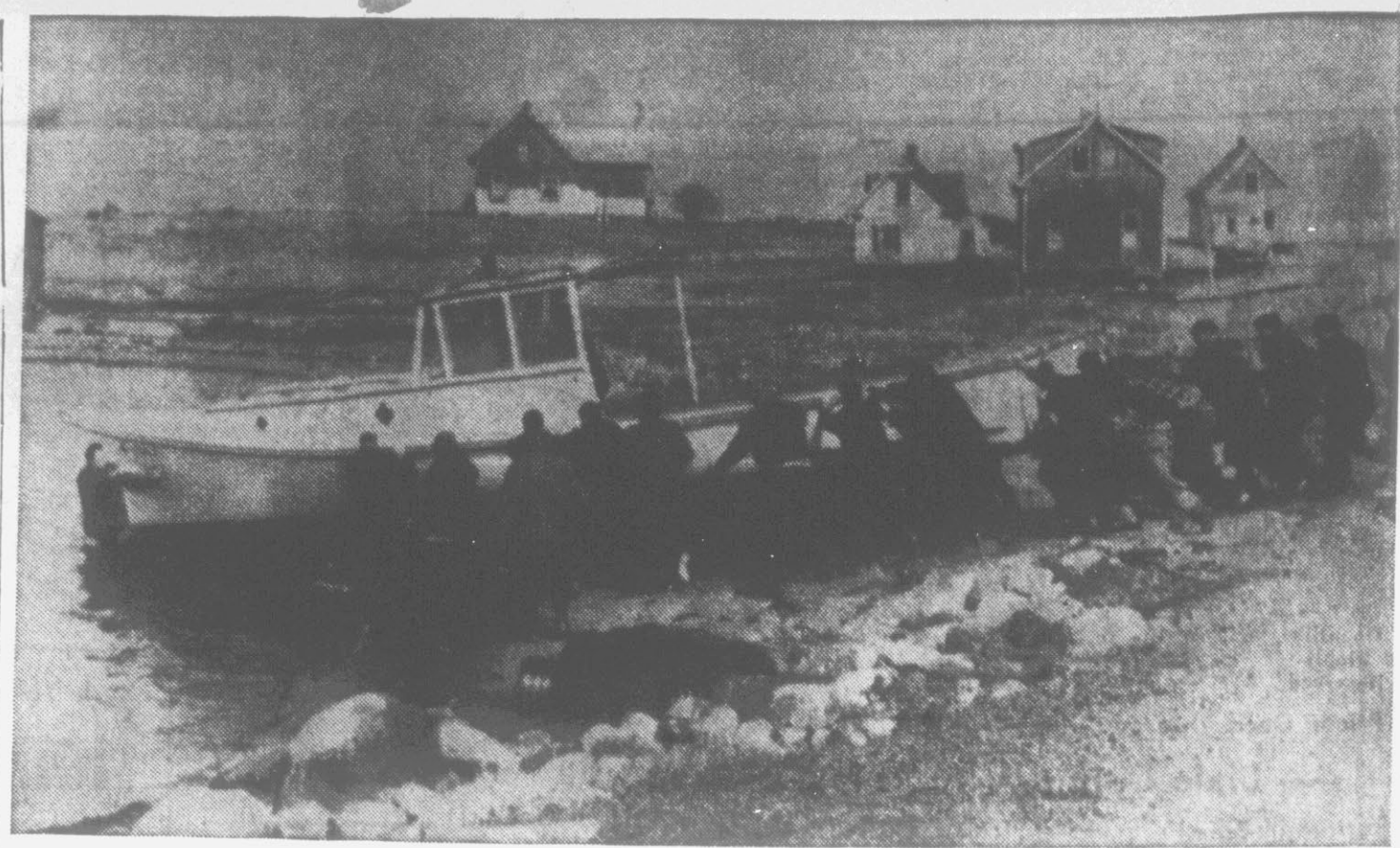
LAUNCHING IN THE DOWN EAST MAINE STYLE — Lobster fishermen of Beals Island, Maine, pool their brawn to launch a 35-footer without benefit of champagne or ribbons. With a shop only a few feet from cove, builder Vinal Beal slides hull bow-first over greased sawmill slabs rather than usual marine railway. Rising tide will float deeper stern free if boat doesn't slide out far enough. (AP Wirephoto)
