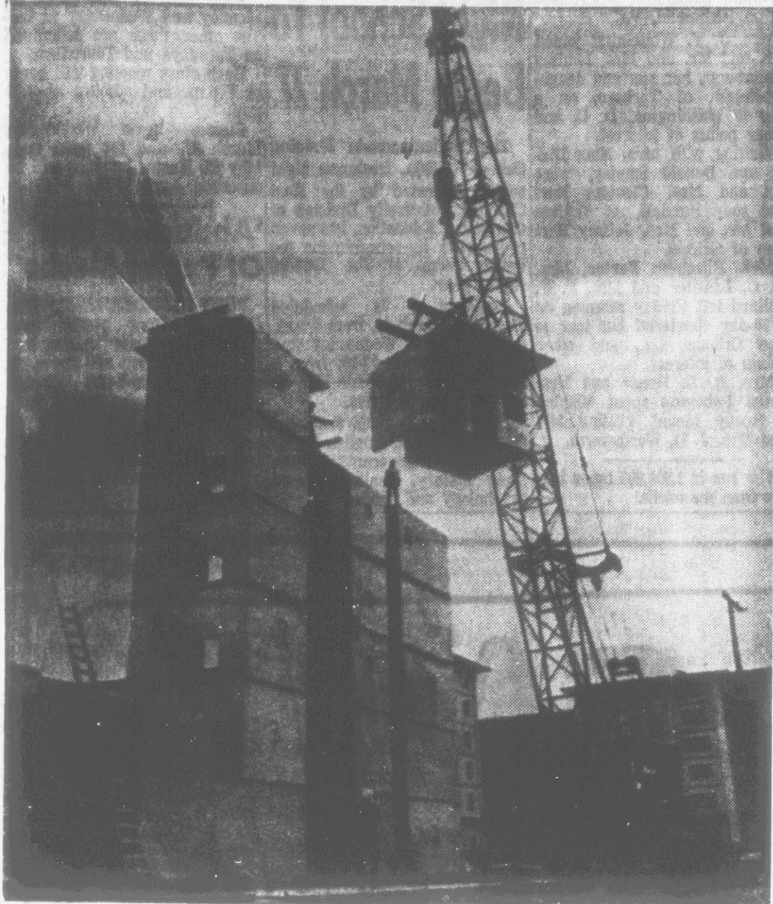
INSTANT APARTMENTS — Cranes lift factory assembled apartment units in place as builders demonstrate fast production in housing in downtown Richmond, Calif. Chemically stressed cement permits three dimensional casting of walls and ceilings in a single unit. The completed structure will be a six-story, 24-unit apartment building. The new technology allows 50 per cent weight reduction thereby allowing economical erection and transportation from factory to job site.
