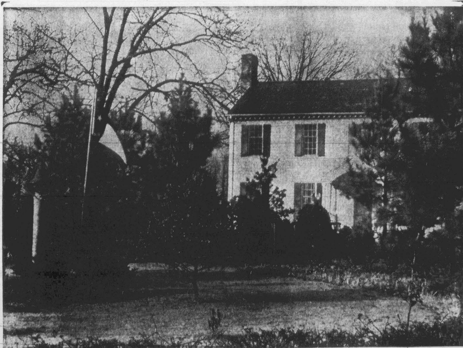
A State Flag flies in the circle drive around the front of Pierce's house. The house itself is filled with antique furniture, civil war relics, replicas of historical state documents and a complete set (over 100 volumes) of the official U.S. Government records of the Civil War.
