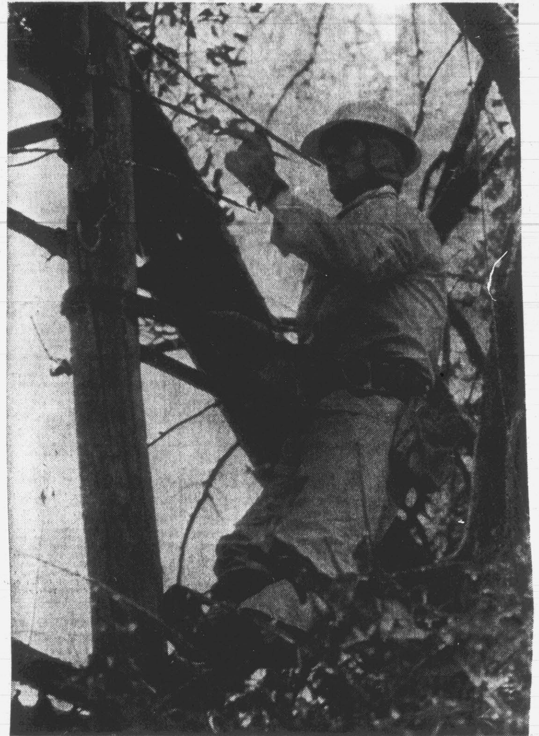
GREENVILLE UTILITIES LINEMAN . . . works atop a pole to replace a power line and restore service in Greenville. (Reflector Photos by Stuart Savage)
