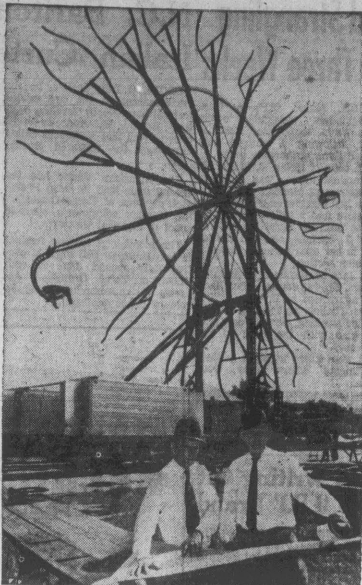
THE FERRIS WHEEL, perennial favorite in amusement parks, has been modified by brothers Elmer Velare (left) and Curtis Velare. Single-arm instead of double-arm support of passenger carriages is intended to give a person the feeling he's in a parachute.
