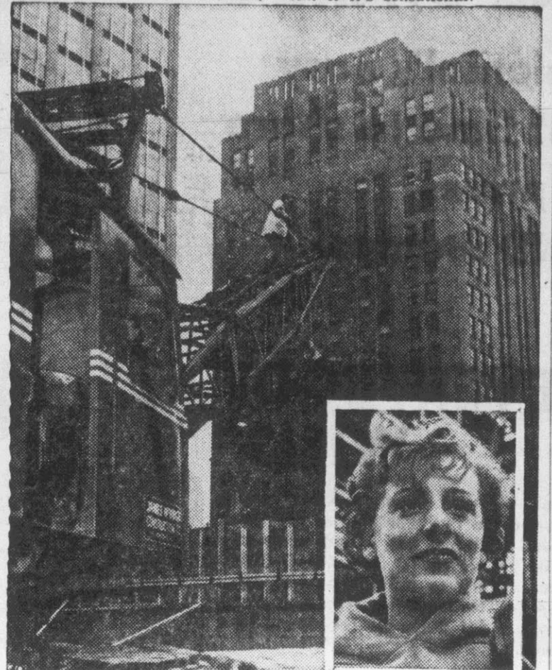
SHE'S ON HER WAY UP . . . Donna Johnson, construction photographer, at work on crane. That's Donna (inset).
