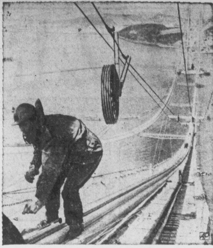
HIGH WIRE MAN —A workman inches up catwalk of Scotland's Forth Road bridge which will be Europe's longest suspension bridge when completed in 1963.
