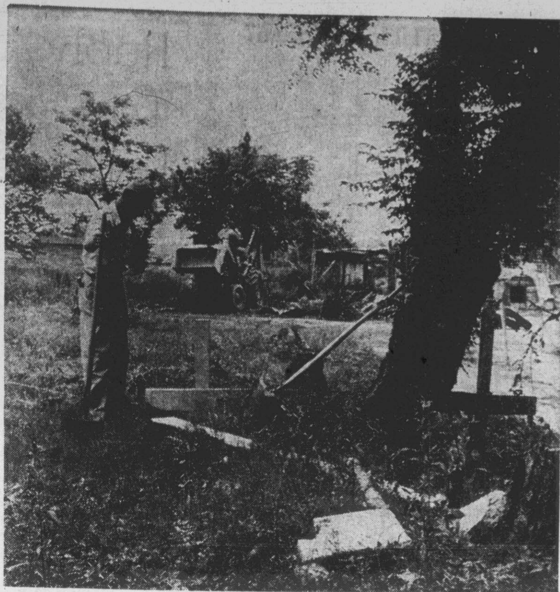
CONSTRUCTION . . . is underway now on a 52,000 square foot plant for Prepshirt Inc., to be located across from the Highway Commission Shops on North Greene St., just outside the city limits of Greenville. Groundbreaking for the new industrial plant was held here last Thursday. The plant, when in full operation is expected to employ about 500 persons.
