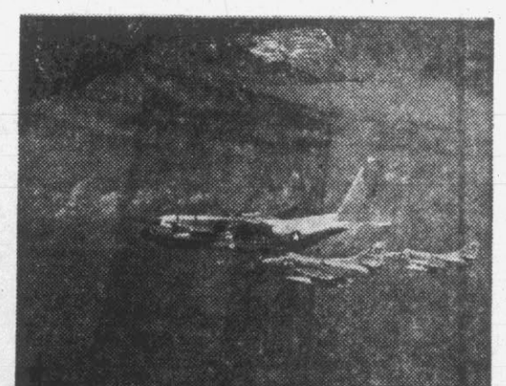
ARMED FORCES DAY 1962 -The United States Marine Corps Lockheed GV-1 Hercules Prop Jet refuels two Douglas A4D Jet Attack Planes.
