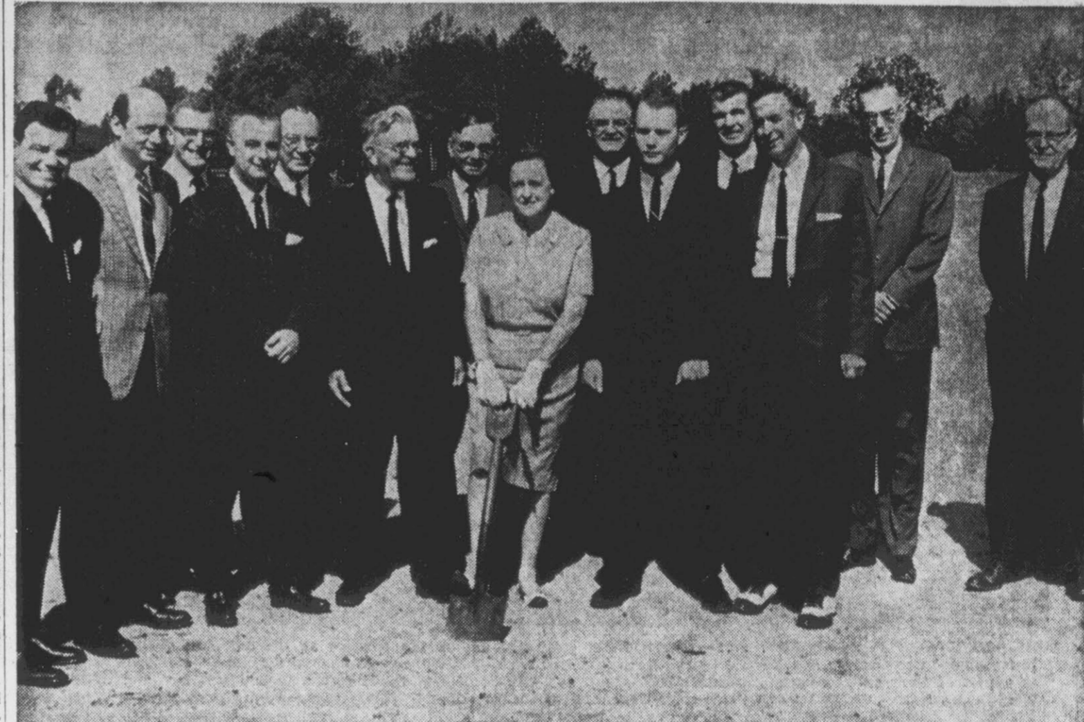
STADIUM CONSTRUCTION UNDERWAY—East Carolina College officials and Stadium Committee members watch as Mrs. James S. Ficklen formally breaks ground with historic spade. From left are Howard, Ficklen, Whickard, Jenkins, Little, Waldrop, Lanier, Mrs. Ficklen, May, Mallison, Hodges, Scales, Duncan and Aycock. (Reflector Staff Photo)
