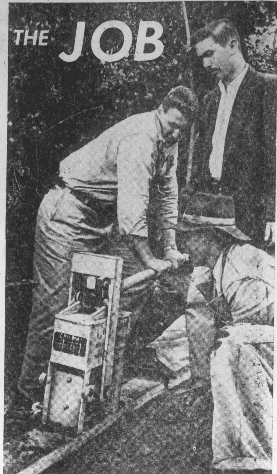
Corpsman George Kroon operates a soil-cement block machine.
