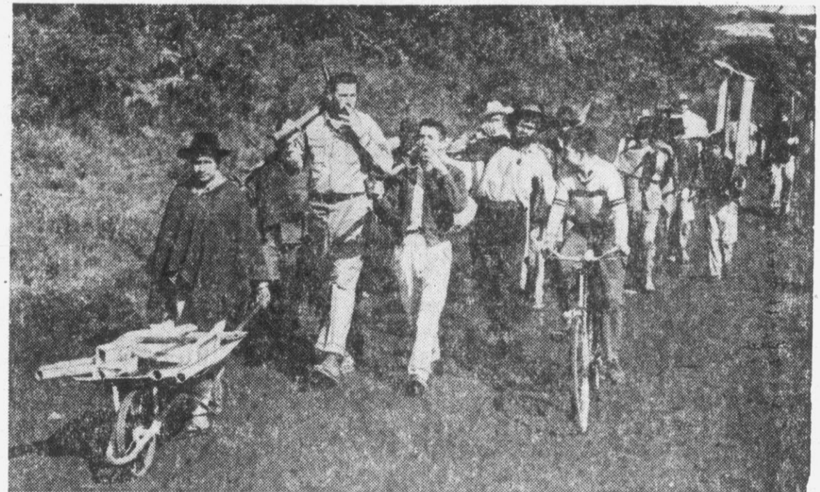
With pick on shoulder, tall George Kroon, in front, marches along with the workers down a dusty road leading to the sand deposit.
