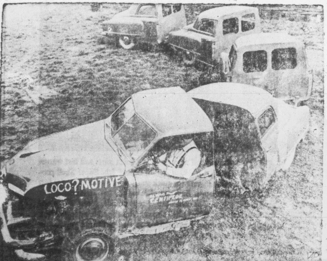
LOCO-?-MOTIVE —Elmer and Ervin Wagner of North Plains, Ore., built this auto train by connecting the rear halves of four scrapped cars to the front half of another car which holds the engine. The power is transmitted to the wheels of each car.
