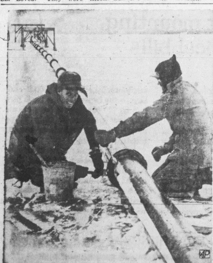
EARLY START —Workmen lay long intake pipe over ice into Lake Champlain for International Girl Scout Roundup camp that opens at Button Bay, Vt., in July.
