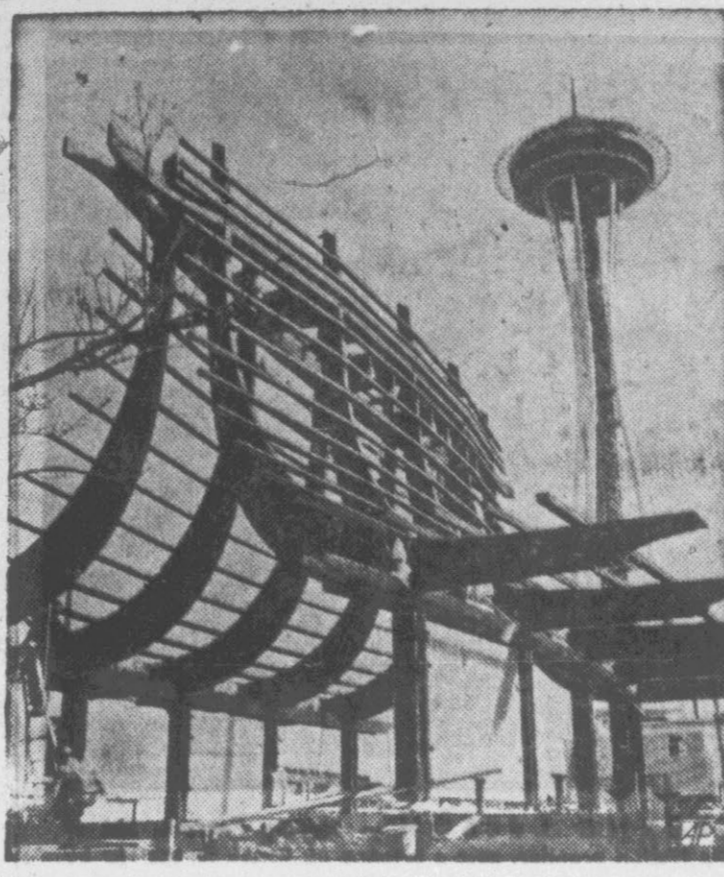
SHAPING UP — Buildings rise on grounds of the Seattle World's Fair. At right is the completed Space Needle, theme structure of the exposition opening in April.
