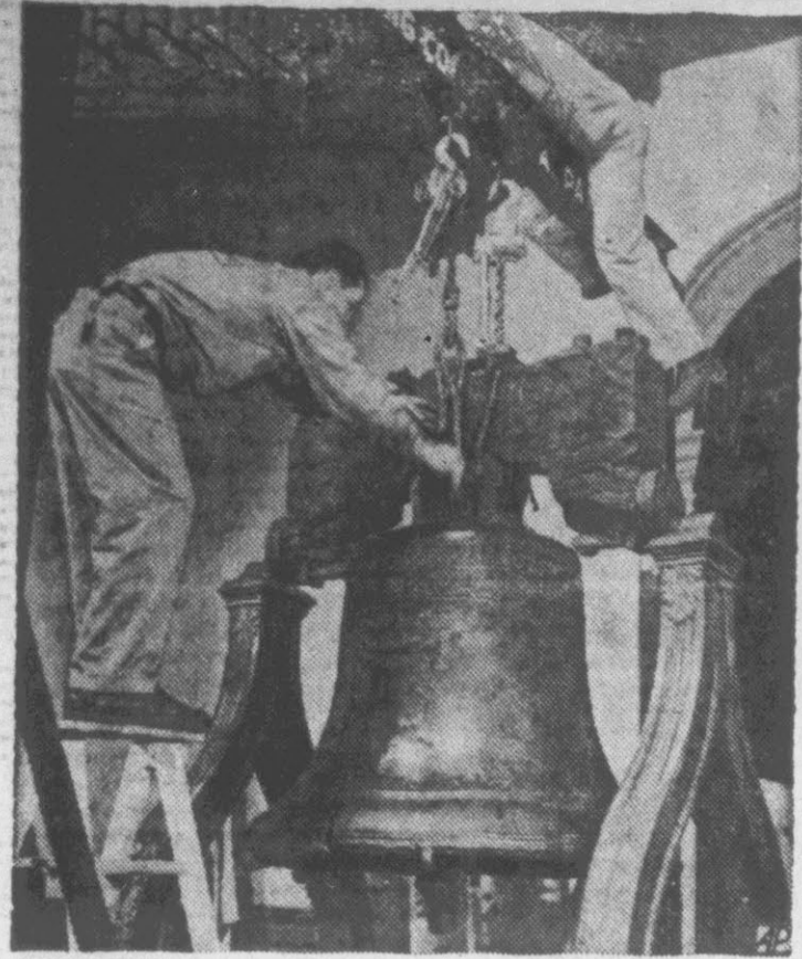
BOLSTER BELL — Workmen raise the famed Liberty Bell in Philadelphia's Independence Hall during delicate task of strengthening yoke from which it hangs.
