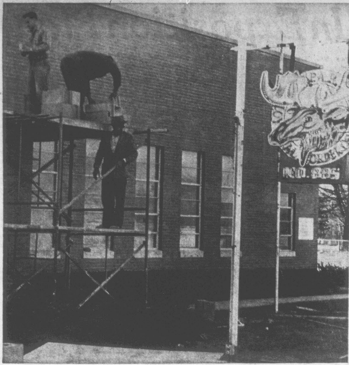
CONSTRUCTION WORK at the Greenville Moose Temple is well advanced on planned remodeling and addition of floor space. The work will result in a new entrance and cloak room, as well as other interior modifications which include expanding the kitchen area. (Photo by S. L. Rowland)
