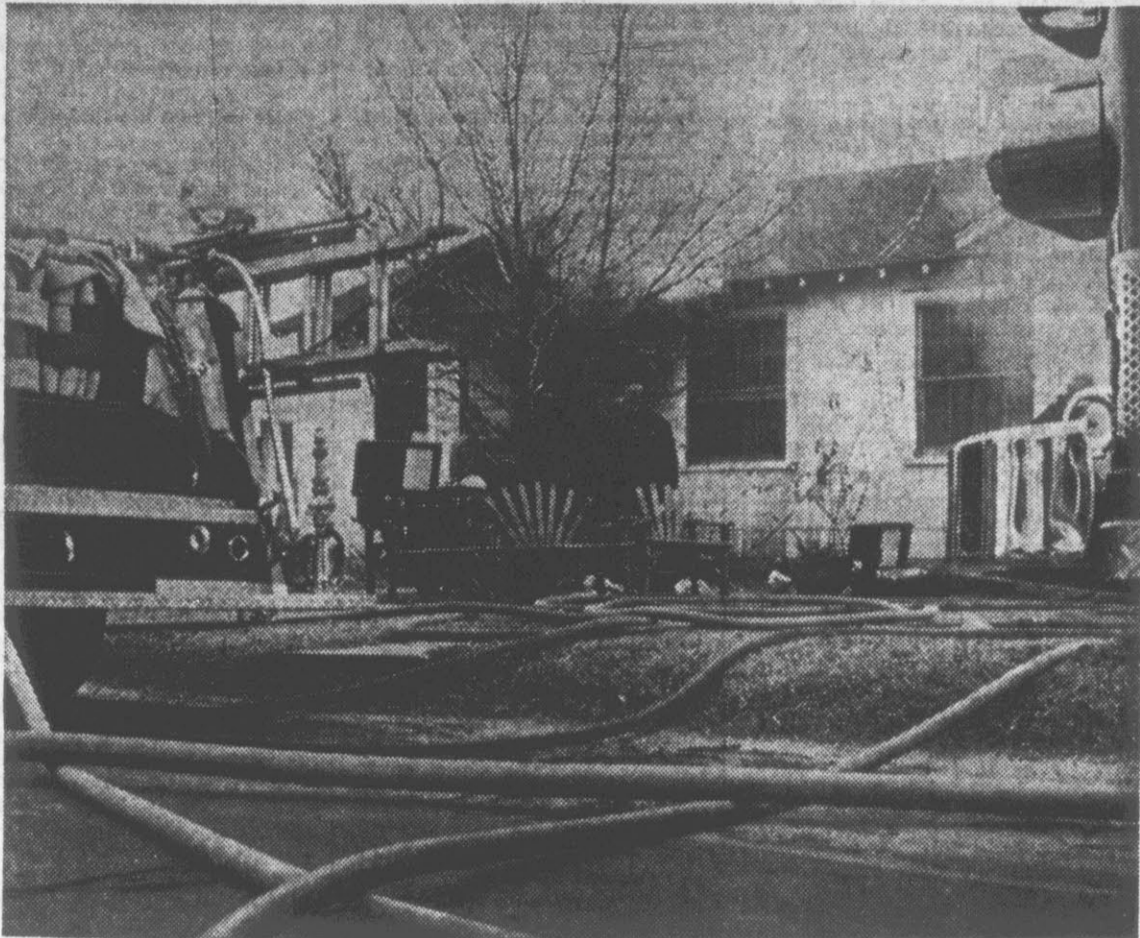
"PEANUTS" IS SAVED . . . as fire guts two rooms in Meadowbrook apartment. (Reflector Photos by Stuart Savage).
