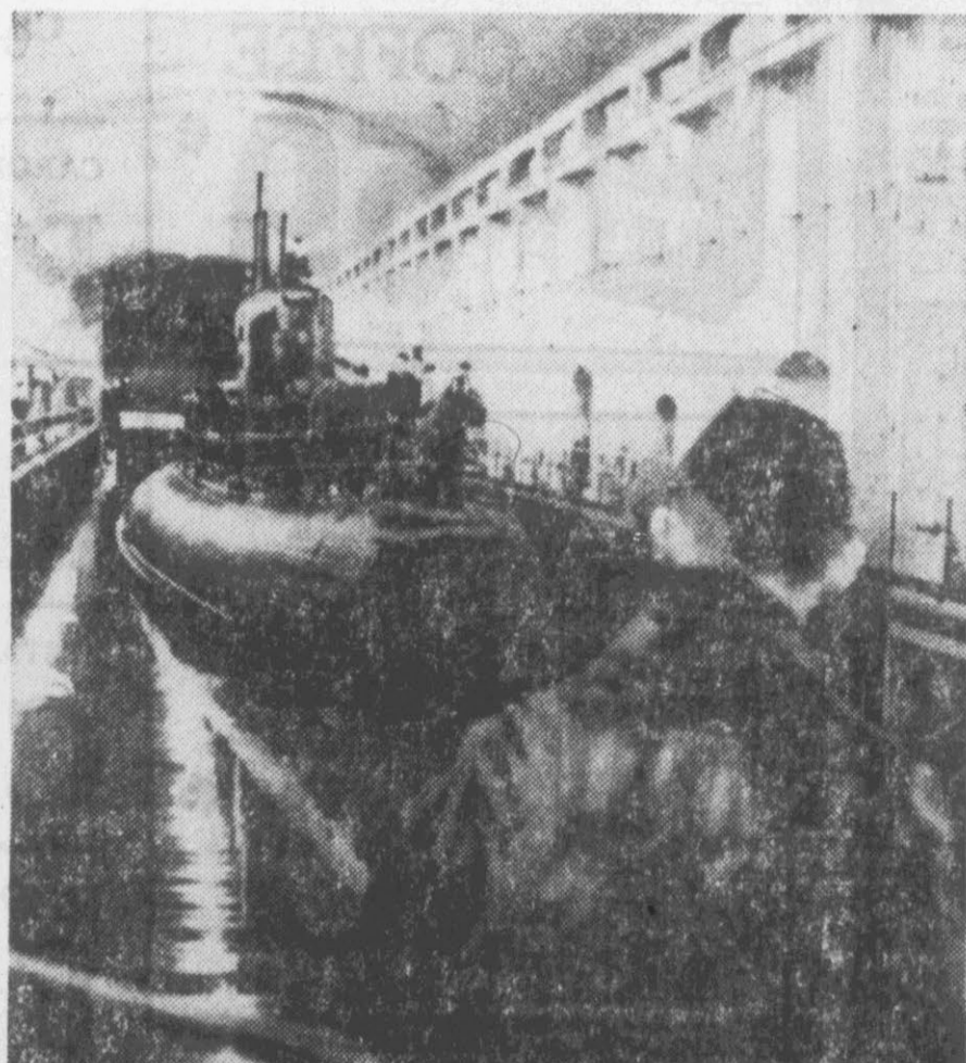
A Swedish Navy submarine is refueled in its underground dock.
