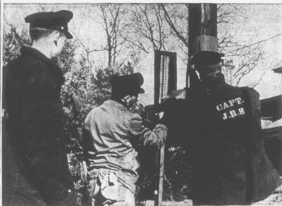
CLEAN-UP TIME . . . These Greenville Firemen are shown as they check out and paint up one of the city's alarm boxes as part of a regular alarm box maintenance program. There are over 110 of these boxes located throughout the city. Pictures are Fireman M. E. Hathaway and Fire Captains, Claude Christopher and Jay Smith.
