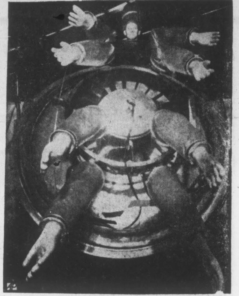
NOT A HALLOWEEN CREATURE —George W. Herren, welder at Tinker Air Force Base at Oklahoma City, peers over his welding blister. The blister is used by Herren in repairing inlet guide vane on the TF-33 turbofan jet engine. The inlet guide vane is the first set of blades which outside air encounters as it enters the engine. A highly toxic gas is created when the blades are heated and the welding blister is placed around the vane assembly. Argon gas is pumped inside. The welder uses the plastic arms to reach various parts of the assembly. (AP Wirephoto)
