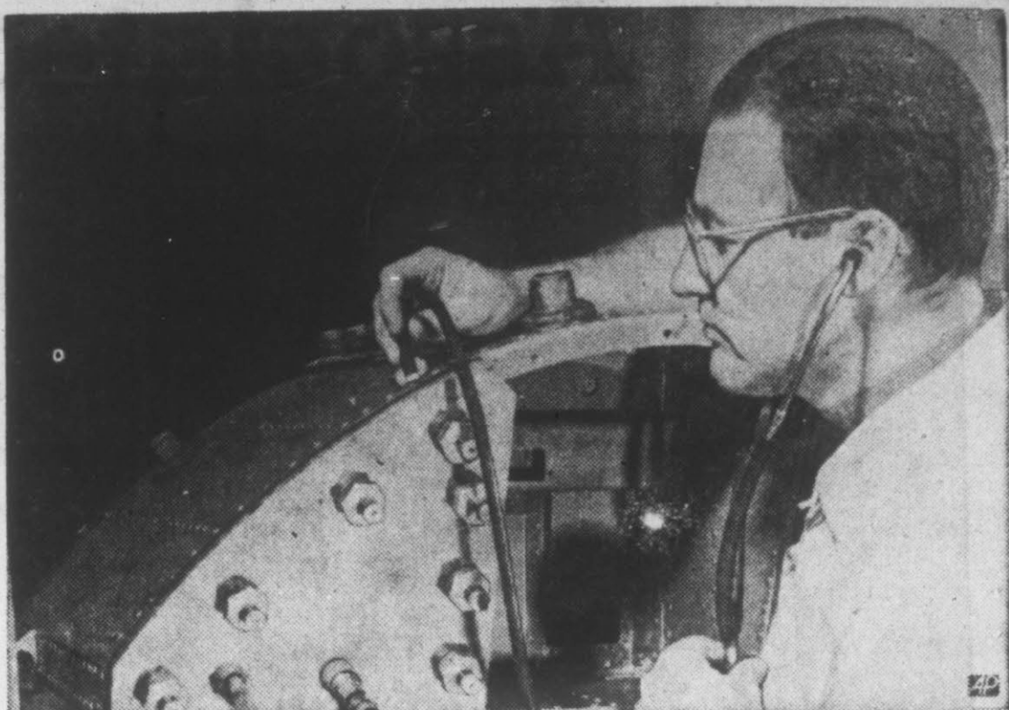
DEFENSE 'DOCTOR' — A technician uses stethoscope to "listen in" for possible leaks in a bombing-navigation console built for the Air Force's B-58 supersonic bomber. Each unit has to be completely sealed to protect the delicate components.
