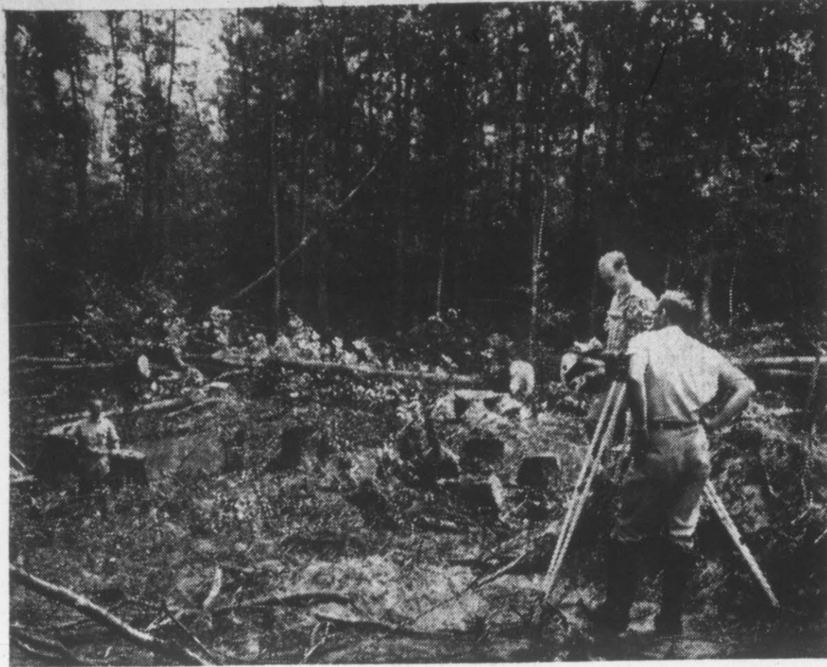
SURVEY PARTY —on Grindle Creek project here stakes for construction on flood control work in Grindle Swamp. Government representative Clifton E. Mills (right) sights through transit to align channel. Amid cypress stumps are Charles E. Godley and Byron Bateman while Hubert Hawkins records survey results. Operation will include use of dynamite to split large stumps in path of proposed channel. (SCS photo by Clifton E. Mills)
