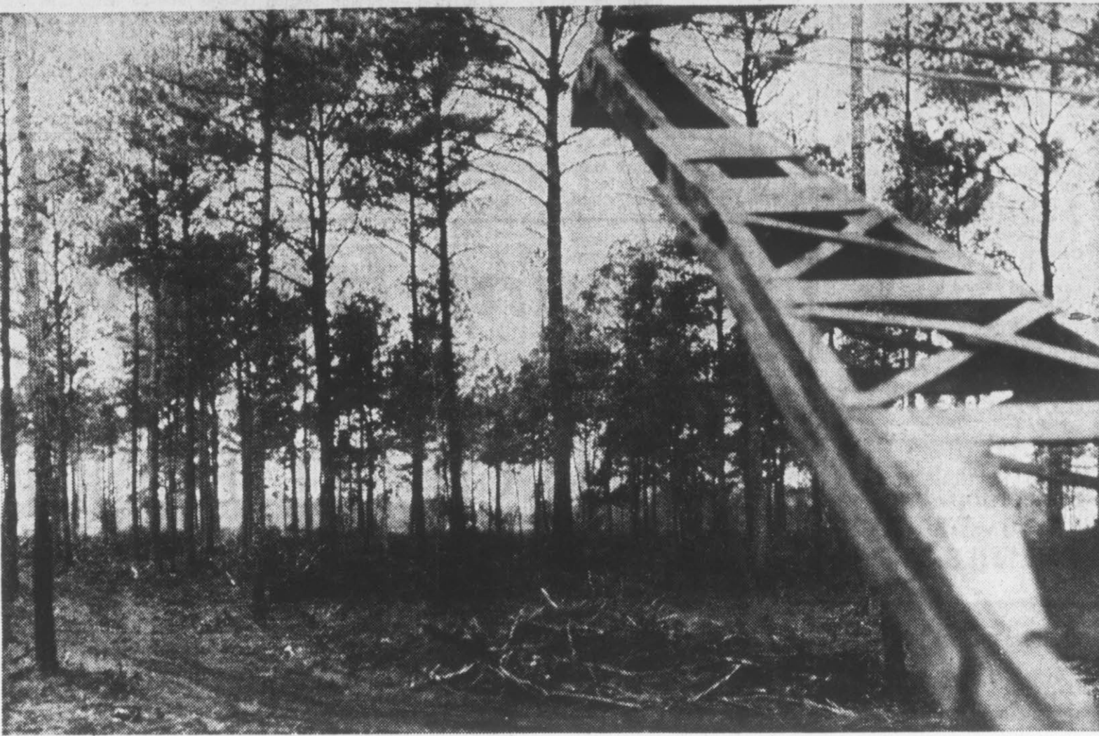
LAND CLEARING FOR INDUSTRIAL SCHOOL . . . site work expected to be completed in ten days. (Reflector Staff Photo)
